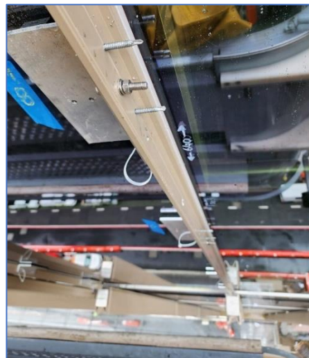
M8 Bolt fixing installed as a secondary measure
