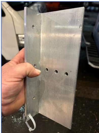
Splice Plate to secure glass panel
