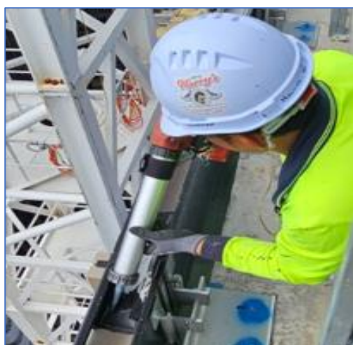
Tether being used to caulk the splice plate.
